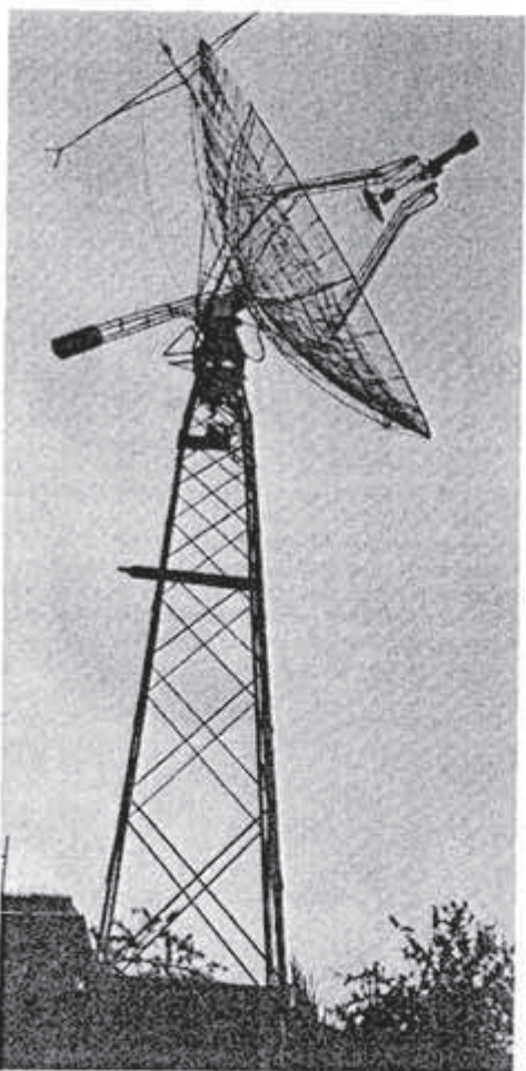
12COR's 8-meter dish for 432 and 1296.
