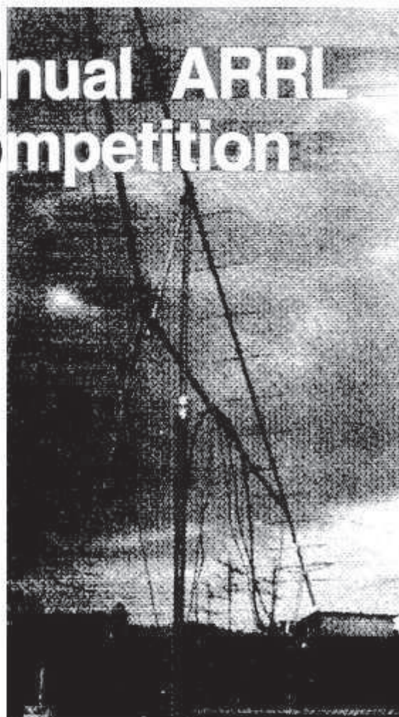
The EME contest doesn't require huge antennas to participate. DL6WU scores very well on 432 using a 24-ft 6-meter-boom single Yagi with an "armstrong" rotator.
