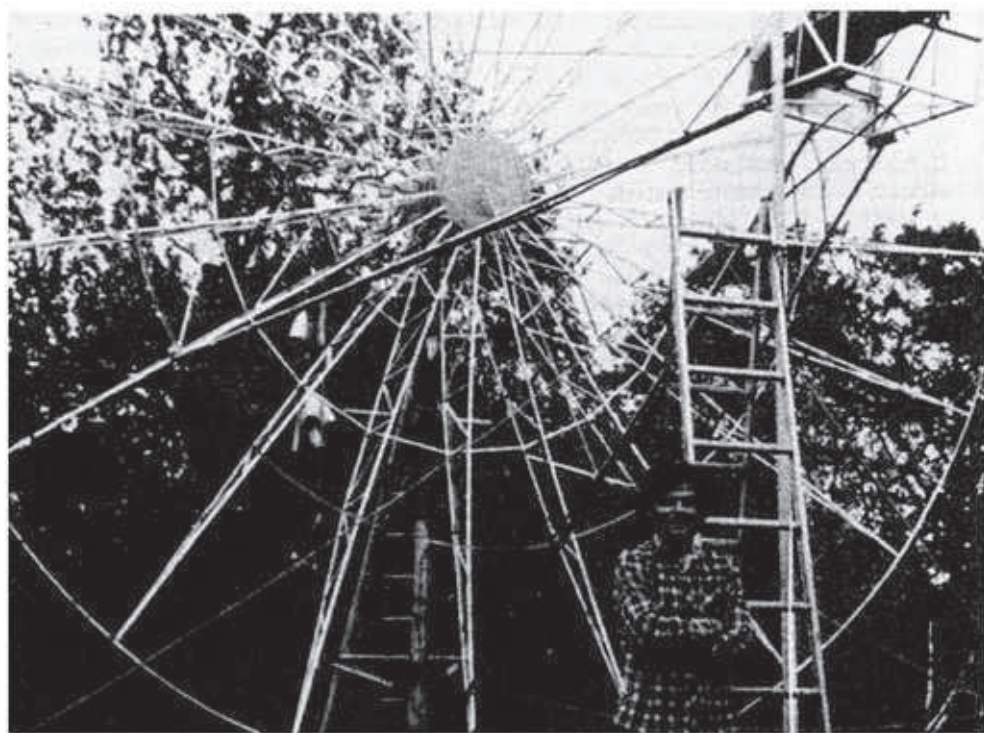
SMØPYP is second only to OE5JFL in the single-operator, multiband category. Paul uses this 7.6-meter dish for 432-2304 MHz.
